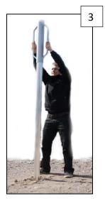
First, make about 40-70 cm (fence with 2 meter posts) or 40-100 cm (fence with 2,3 meter posts) deep holes to the ground for the corner posts with a power drill or pinch bar (1). Depth depends on the fence model and the quality of the soil. Put the nylon cover on the top of the post before hammering.
